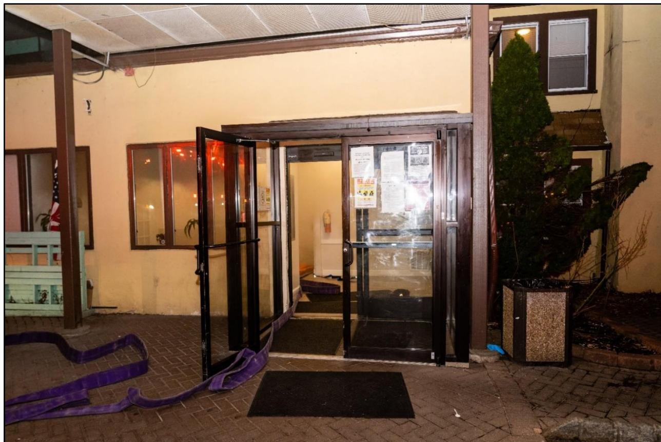
Photo 4. Photograph of smoke condition observed in the lobby. The 3-inch hoseline from Tanker 17 was stretched up the stairwell to the 2 nd floor. The time was approximately 01:12 hours.
